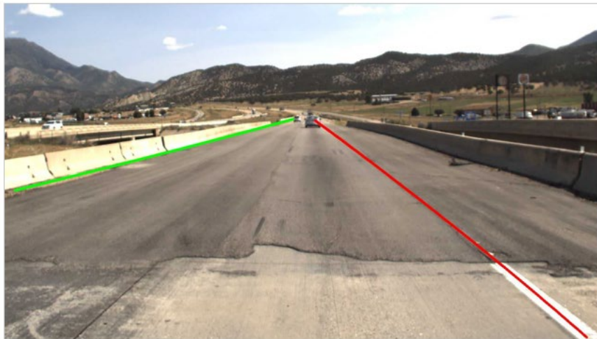
Missing Marking on Resurfaced Overpass
